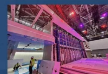
搭建现场 Build the site
