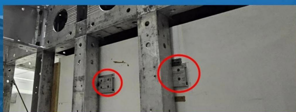
挂板扣件与效果 / Hanging board fasteners and their effects
