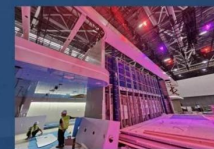
搭建现场 Build the site
